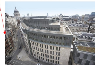
St Bartholomew's Hospital, London, Opened in June 2016
